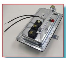
If both HOT and NEUTRAL are available, wire the lamp parallel with the load for ON indication or on the opposite contact for OFF indication.
