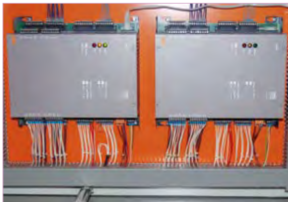
Control cabinet before and after conversion: the existing Staefa controller is on the left, the Saia-Burgess Controls conversion set with PCD2.M5540 is on the right
