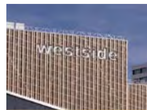
Shopping- and Leisure centre Westside 66
